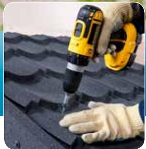
Made from lightweight high grade steel with Aluzinc® coating for incredible strength and weather protection
